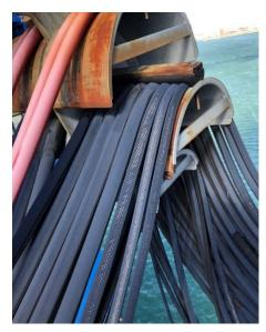
Photo above shows a portion of festoon cable system. Note deterioration of outer jacket.
