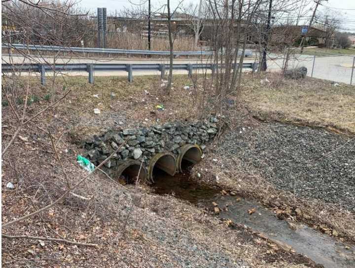
Photo 49: Atlantic Ave. headwall, south of Atlantic Avenue, looking north.
