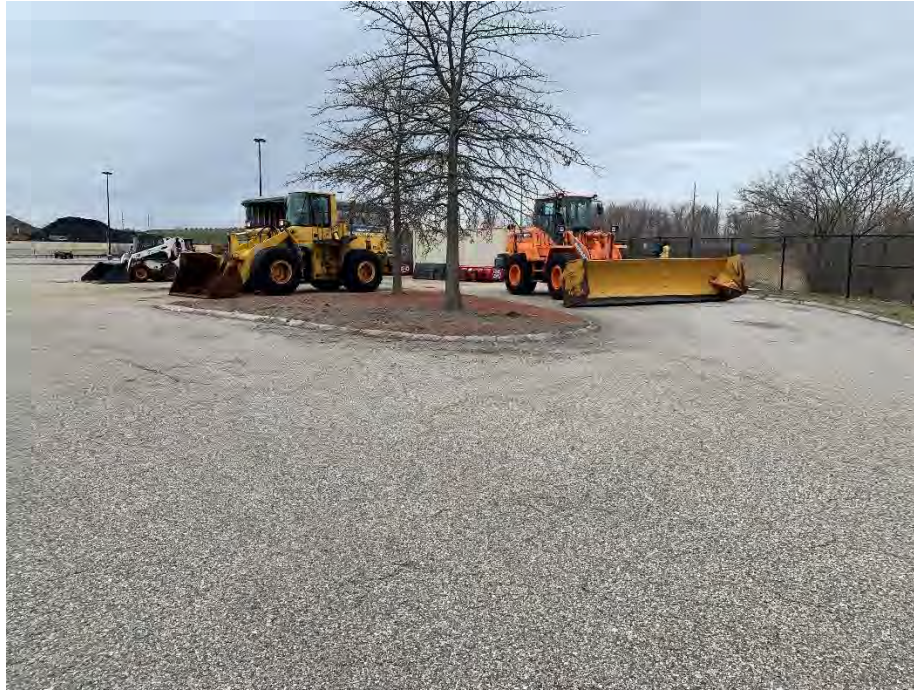
Photo 9: Observed minor cracking (near northeast entrance), looking west.
