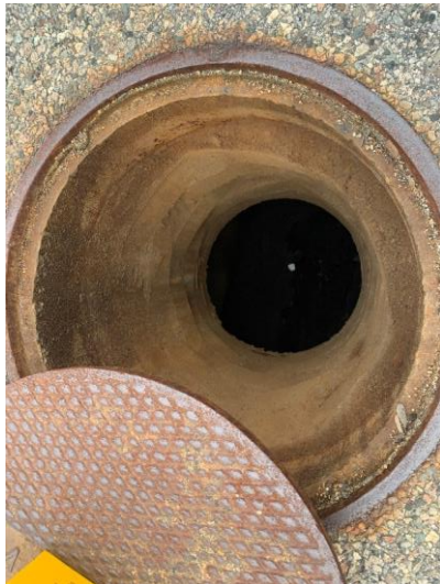
Photo 4: MH10 appears to be in good condition.
