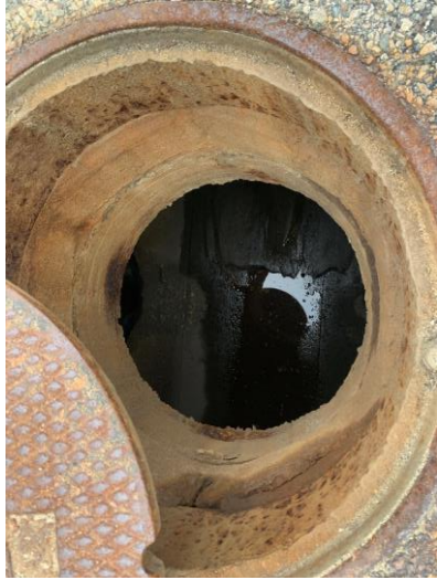
Photo 5: MH15 appears to be in good condition, <1 inch of sediment accumulation.
