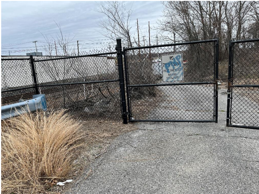
Photo 12: Top rail disconnected, near SF-6, looking north.
