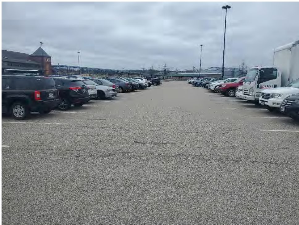
Photo 42: Observed minor cracking in the pavement in the north section of the commuter rail parking area, looking west.
