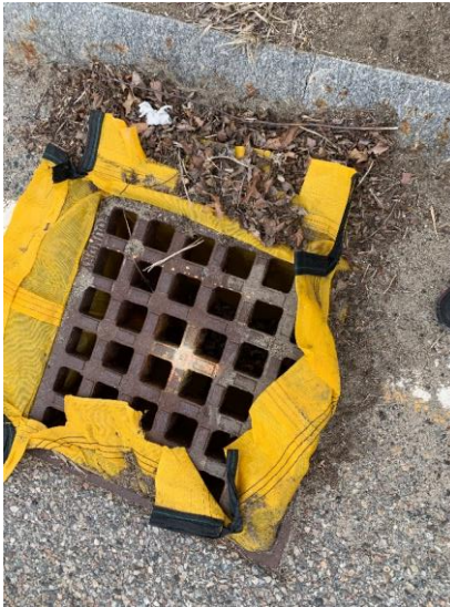
Photo 42: CB30 contained a silt sack with minor accumulation of organic debris.
