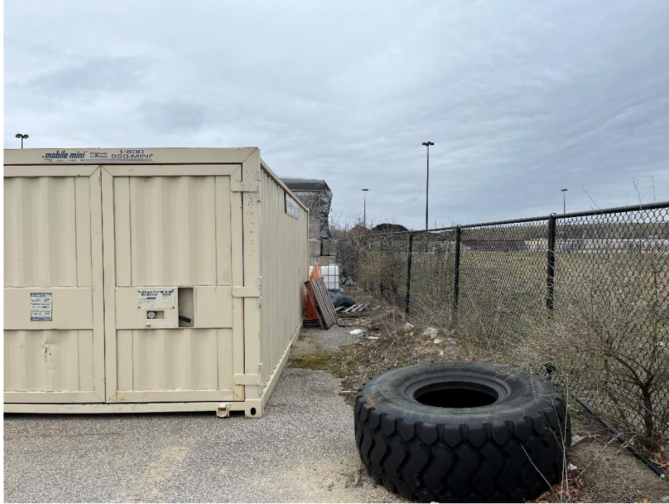
Photo 1: Vegetation and bowed fabric, looking northwest near sand shed.
