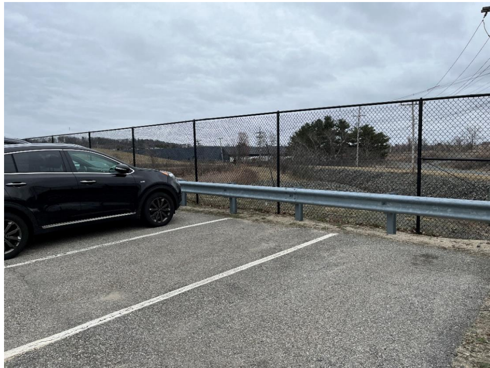
Photo 22: Warped fabric, disconnected fabric, the southern edge of the site, looking south.
