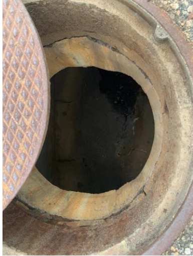
Photo 3: MH3A appears to be in good condition.
