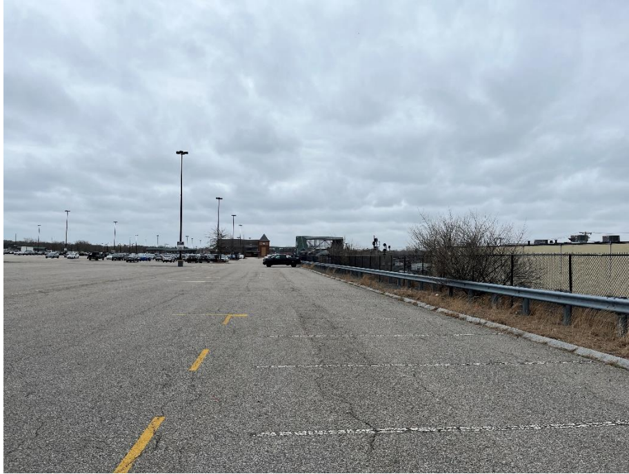
Photo 5: Gravel covering along west, center side of commuter rail parking lot near MBTA tracks, looking southwest.
