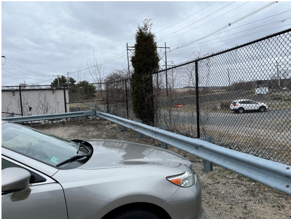
Photo 20: Vegetation growing through fence fabric along the southern edge of the site, looking south.
