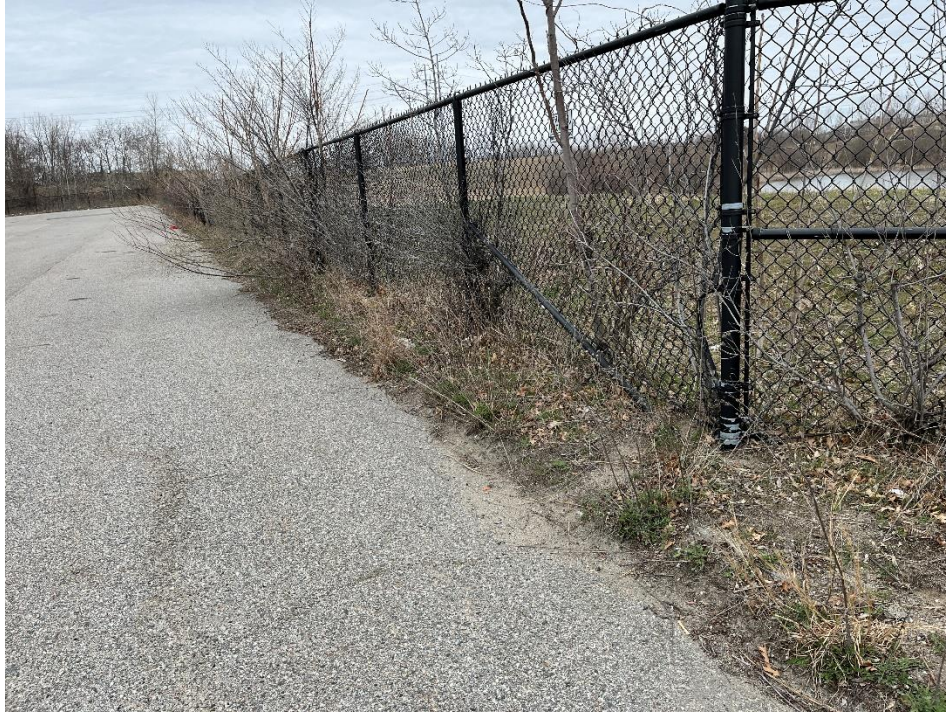
Photo 3: Vegetation growing through fence fabric and hole in the fence, looking northwest.
