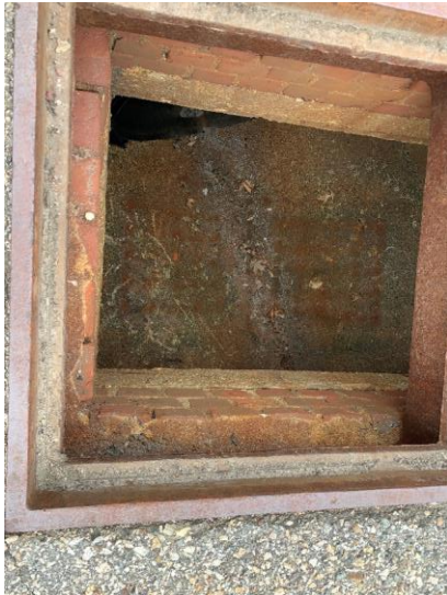
Photo 38: CB26 in good condition, no sediment accumulation observed.
