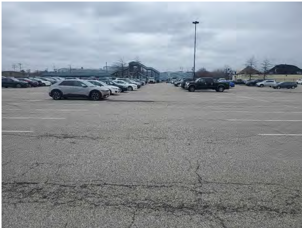
Photo 30: Observed moderate/severe cracking in the pavement in the north section of commuter rail parking area northwest of GB964, looking west.
