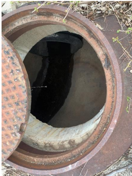
Photo 8: MH34 appears to be in good condition.
