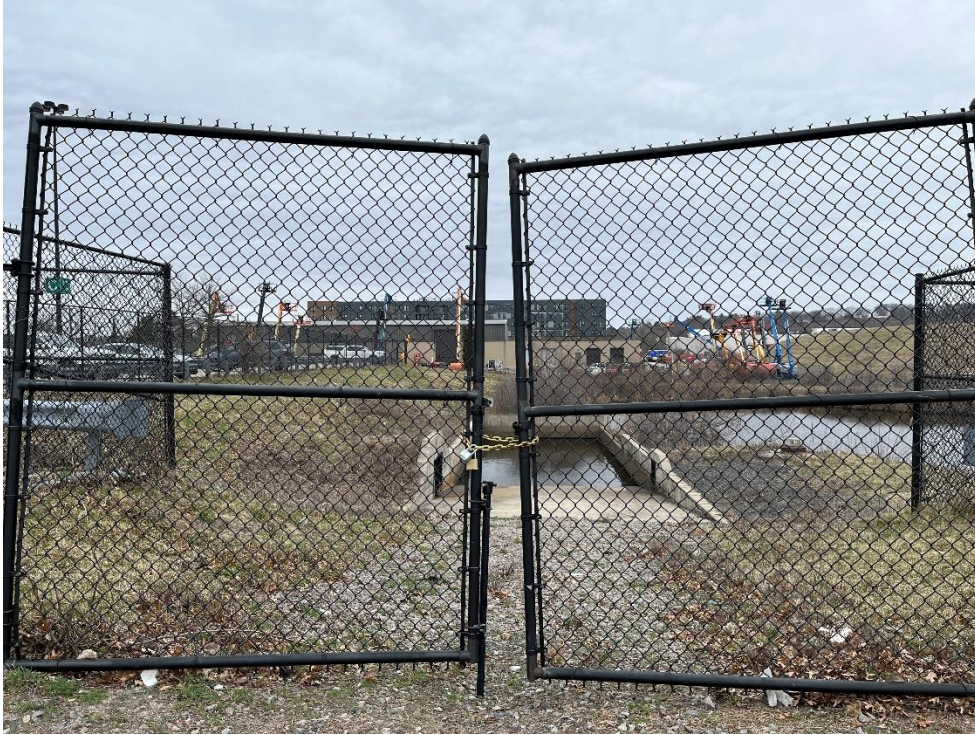
Photo 23: Damage to a gate near the southwest corner of the site, hinge appeared damaged, looking southwest.
