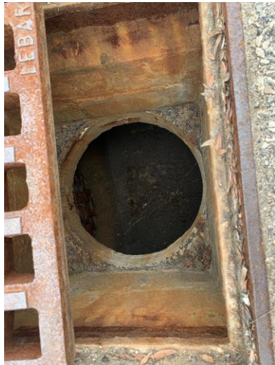
Photo 16: CBSA appears to be in good condition, no sediment accumulation observed.
