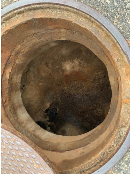
Photo 9: MH102 appears to be in good condition, <1 inch of sediment accumulation.
