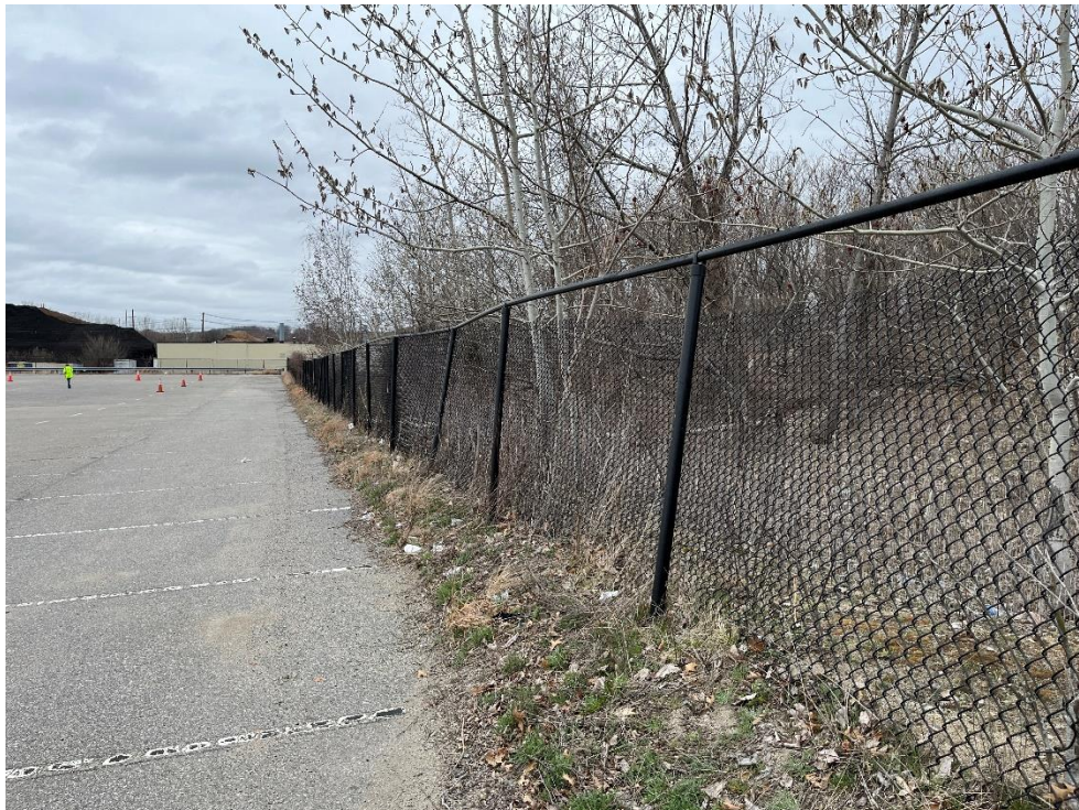
Photo 8: Bowed fence fabric near SF-5, looking west.
