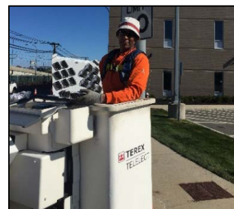
Retrofitting streetlights with LEDs
