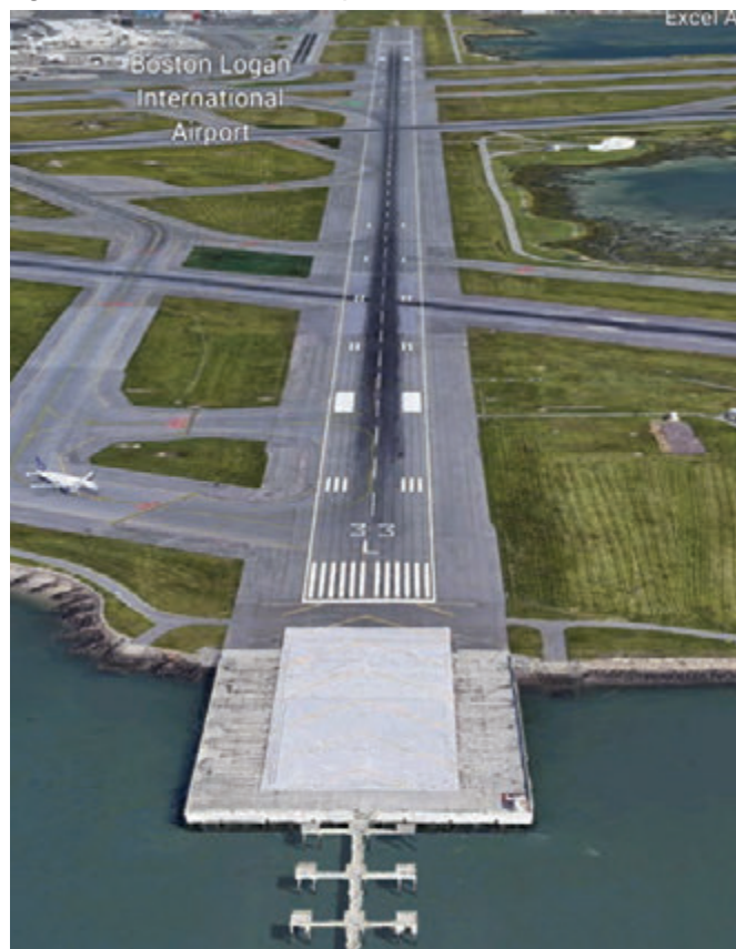
The EMAS at the east end of Runway 33L
