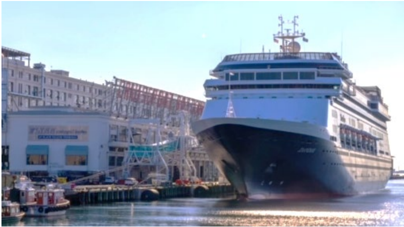
Cruise Terminal Seawall Structural Rehabilitation
