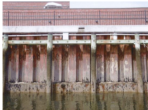
Steel Sheet Pile
