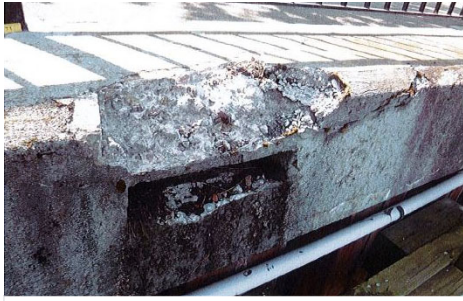
Concrete Spall
