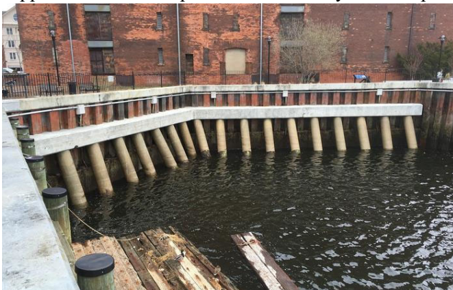
Steel bulkhead with concrete girdle and batter piles
