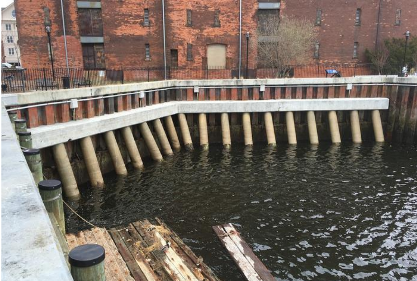
Steel bulkhead with concrete girdle and batter piles
