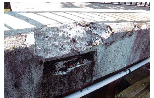
Concrete Spall
