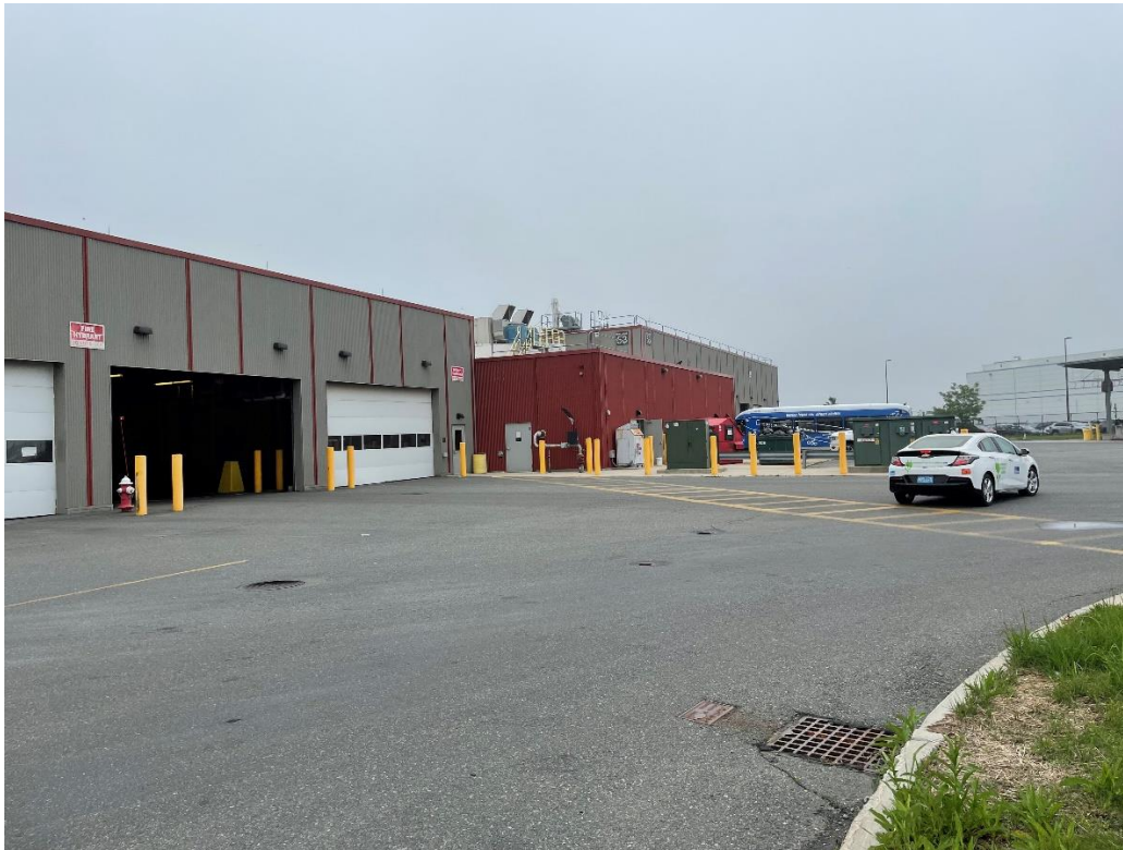
Figure 3: Existing GBD Maintenance Bays, Main Entry & Cold Storage
