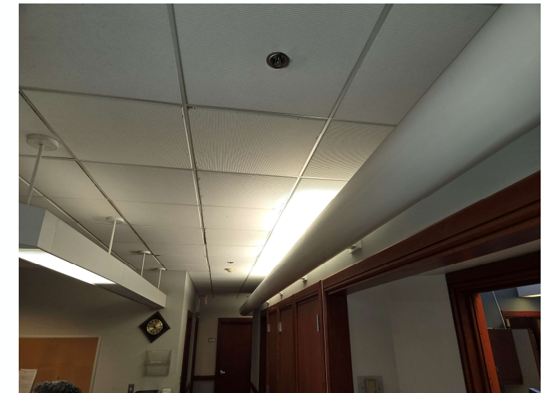
Facilities I Administration Building (L018)
