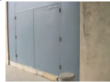
Eversource & MPA Electrical
