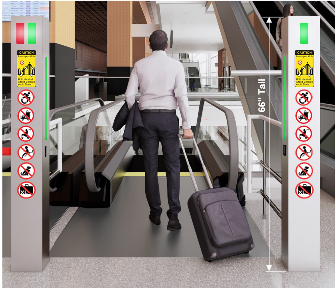
Figure 13: View of a typical pair of escalator pylons showing the caution and safety signage.
