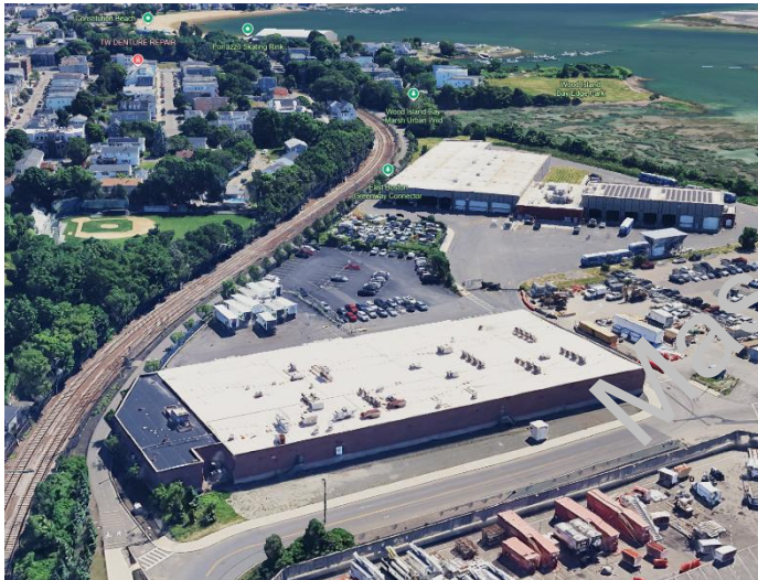
Existing Condition Aerial View
