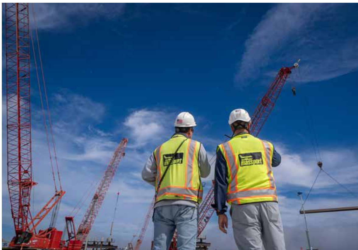
BOS Logan Airport Runway construction project.
