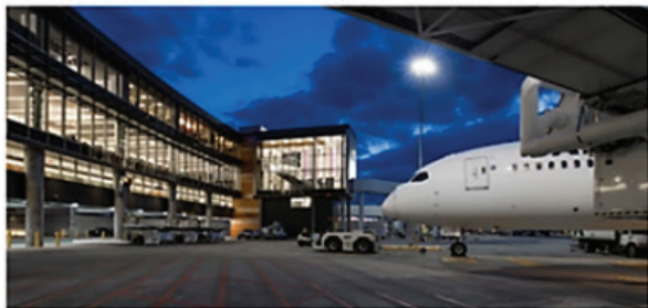
FIGURE 3 — Terminal E Crescent
