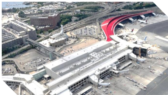
Figure 2- Terminal E Logan Airport
