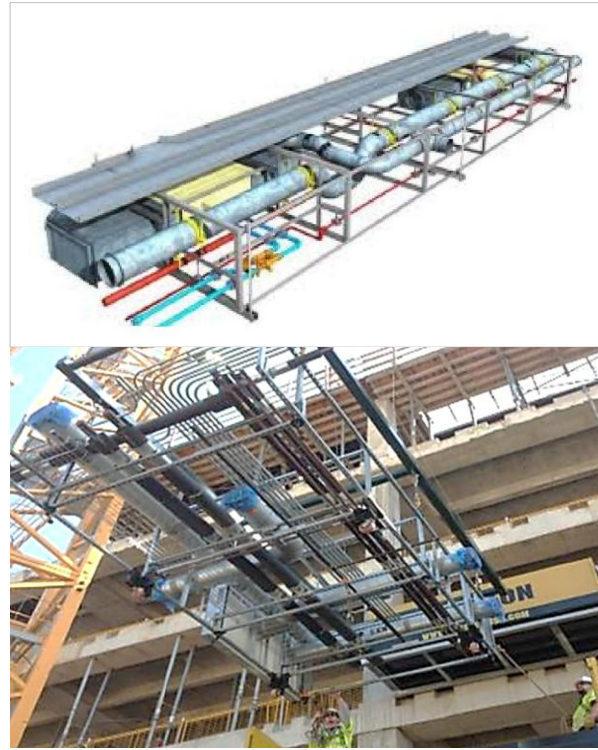
Figure 82- Prefabrication Model Installation
