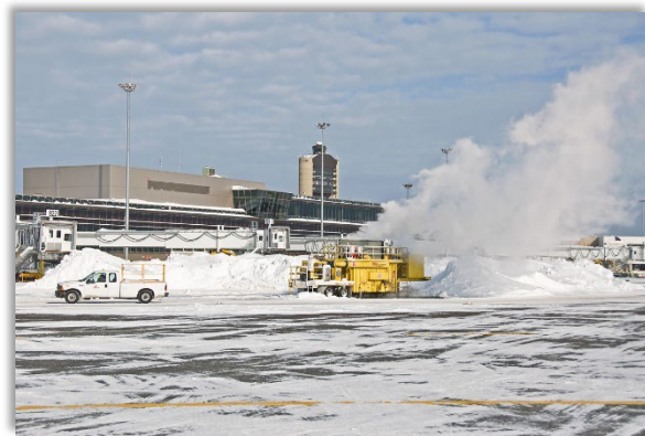
Snow Melter at Logan Airport.
