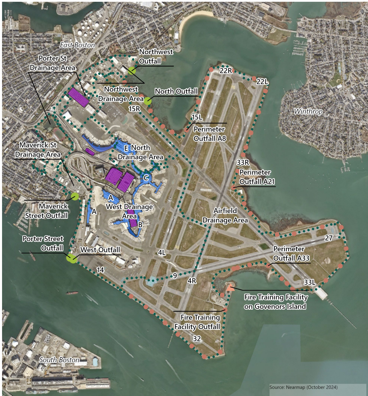
Figure 9-1 Logan Airport Outfalls
