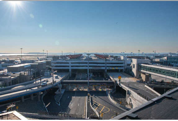
Terminal B Garage.
