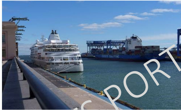
Cruiseport Pier Rehab (on-going)
