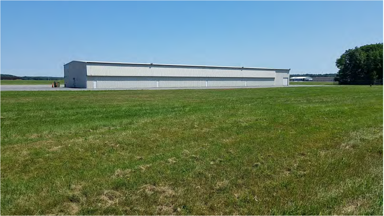
Photo 3: View of an existing t-hangars building at Pine Hill Area.
