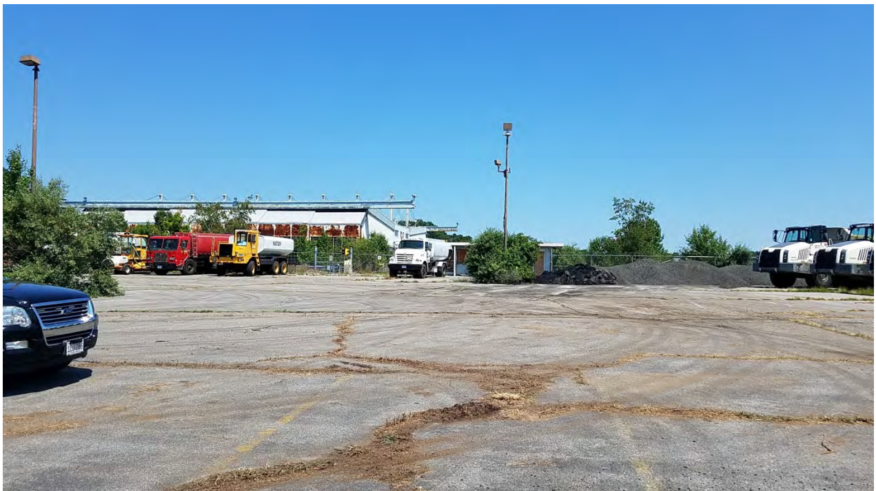
Photo 6: Existing paved areas at the North Airfield Area looking east.
