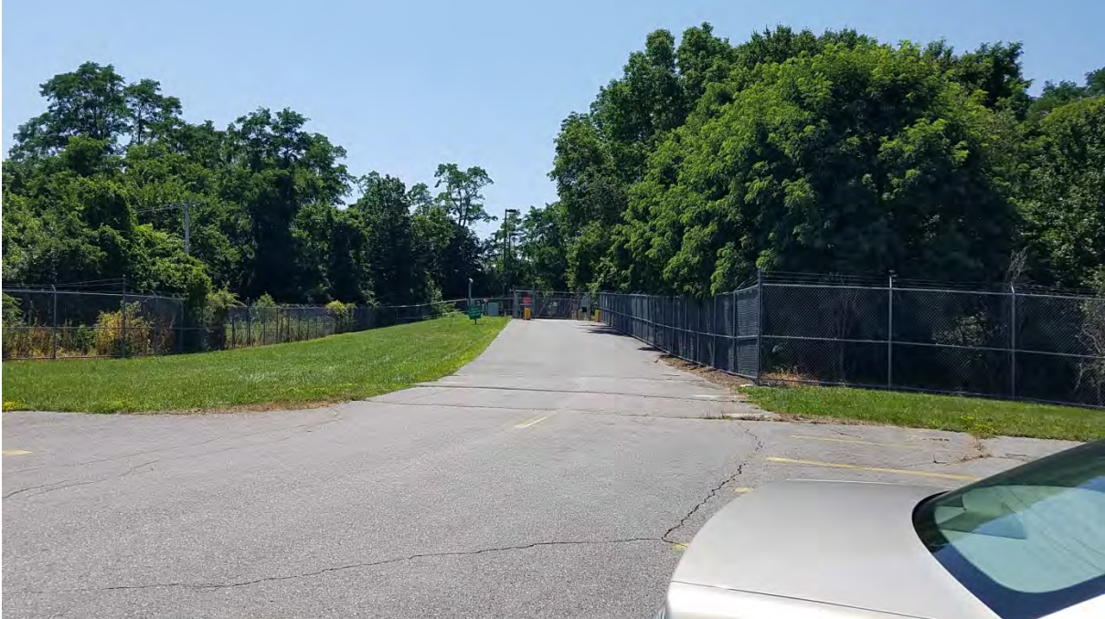
Photo 2: View of access to Virginia Road at Pine Hill Area
