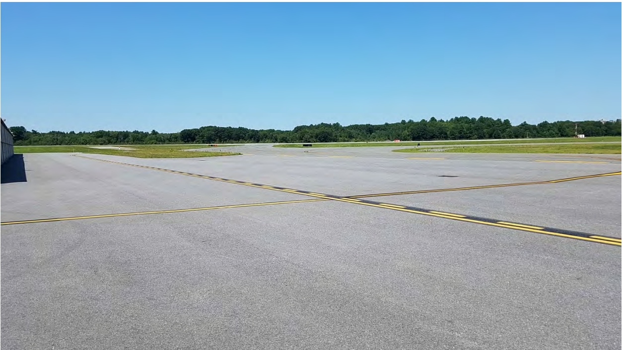
Photo 4: Existing apron space at Pine Hill Area.
