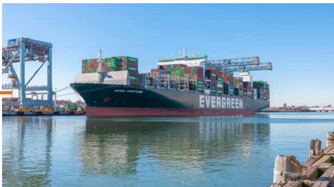
Evergreen's Ever Fortune at Conley Container Terminal
