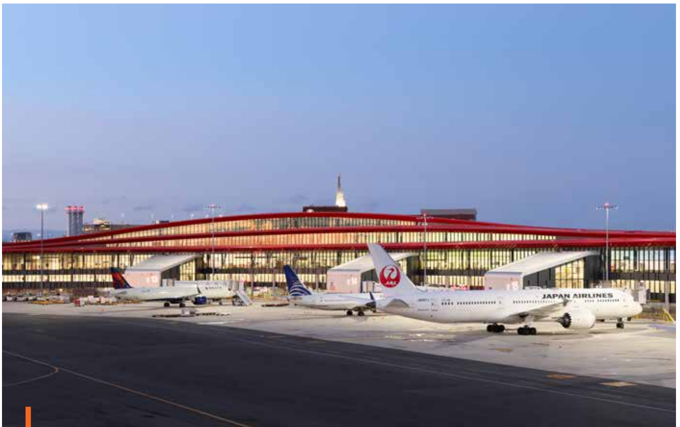
View of modernized Terminal E and new aircraft gates from the airfield.
