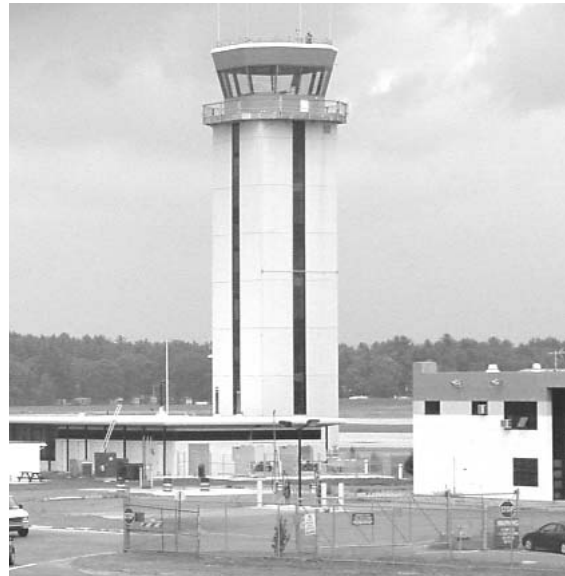
New FAA Air Traffic Control Tower.
